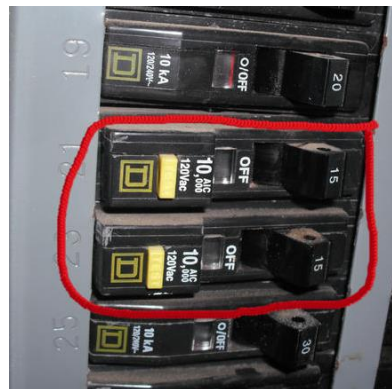
GFCI Breakers
